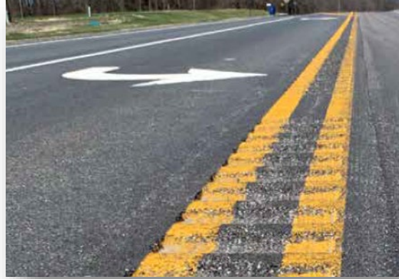
R30- Install centerline rumble strips/strips
