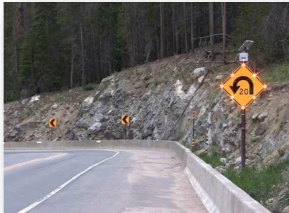
R24- Install curve advance warning signs
