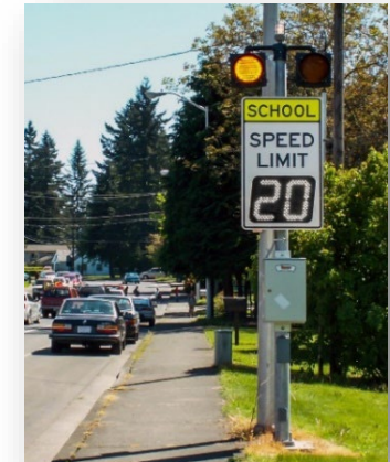
R26- Install dynamic/variable speed warning signs
