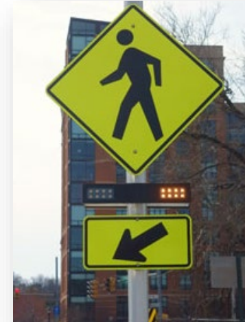
R38PB- Install Rectangular Rapid Flashing Beacon (RRFB)
