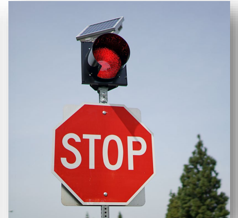
NS11- Install flashing beacons as advance warning (NS.I)
