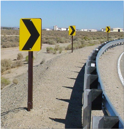
R23- Install chevron signs on horizontal curves
