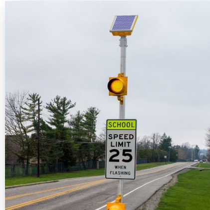
SI09- Install flashing beacons as advance warning (S.I.)
