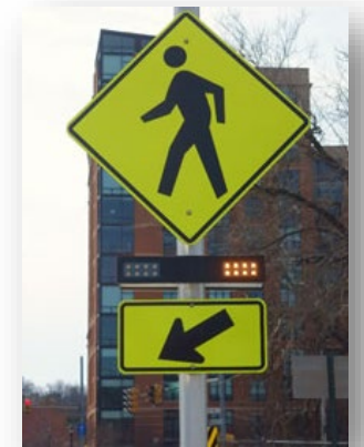
NS24PB- Install Rectangular Rapid Flashing Beacon (RRFB)
