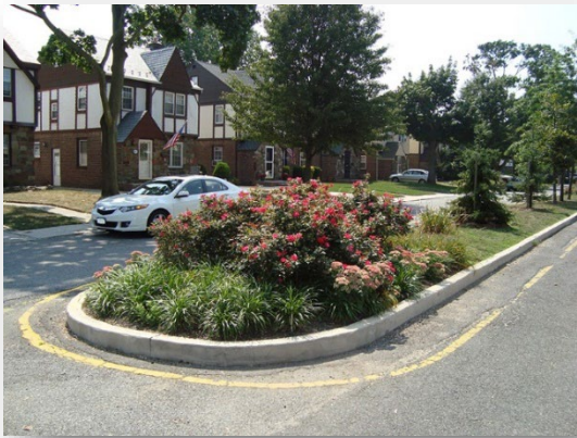
NS16- Install raised median on approaches (NS.I.)
